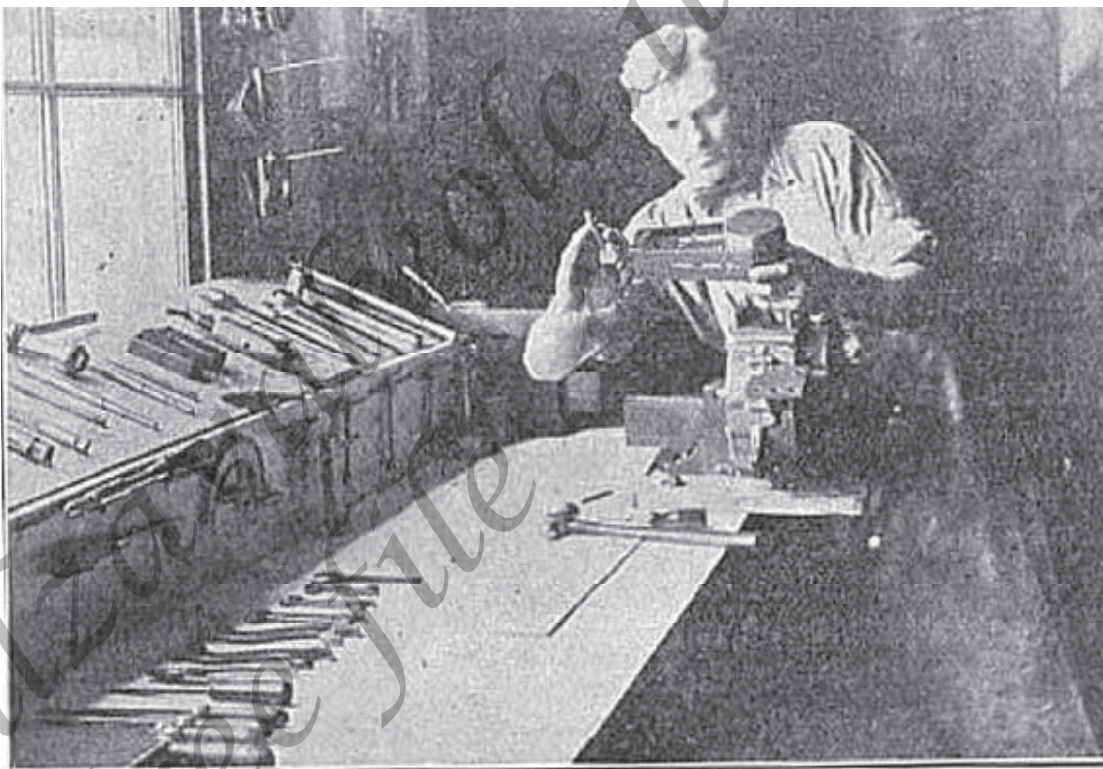
Fig. 356.—How to Remove Harley-Davidson Wristpins from Pistons
